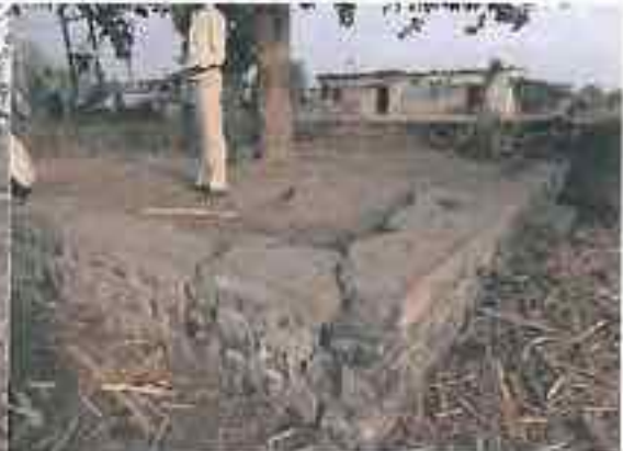
Ratwa: Two platforms, one with lots of vegetation and shrubs: Improper filling, poor maintenance; another has a damaged structure with wide cracks.
