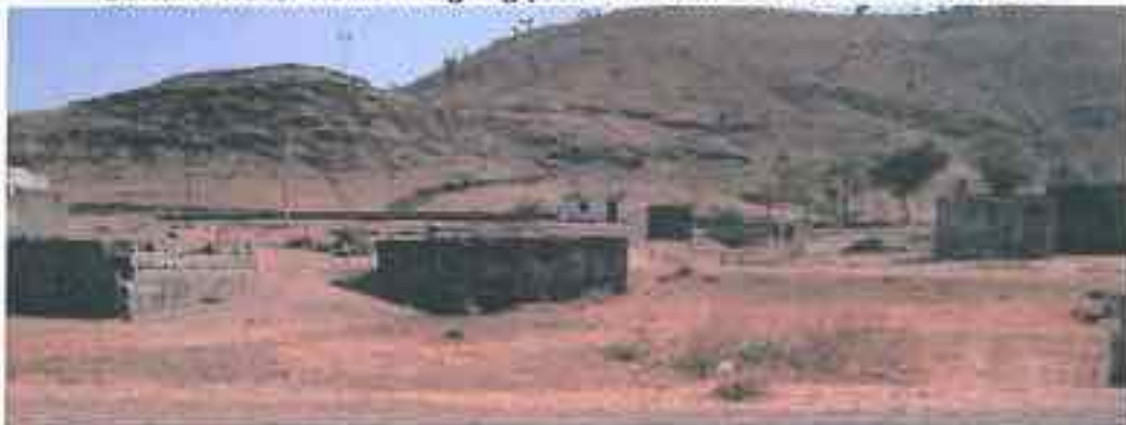
Borlai II: Another set of culverts-water from hills left free to zig-zag
