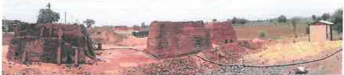
Plate 3.1.47. Tawlai Khurd: Brick making next to public TW, making it defunct (Typical)
