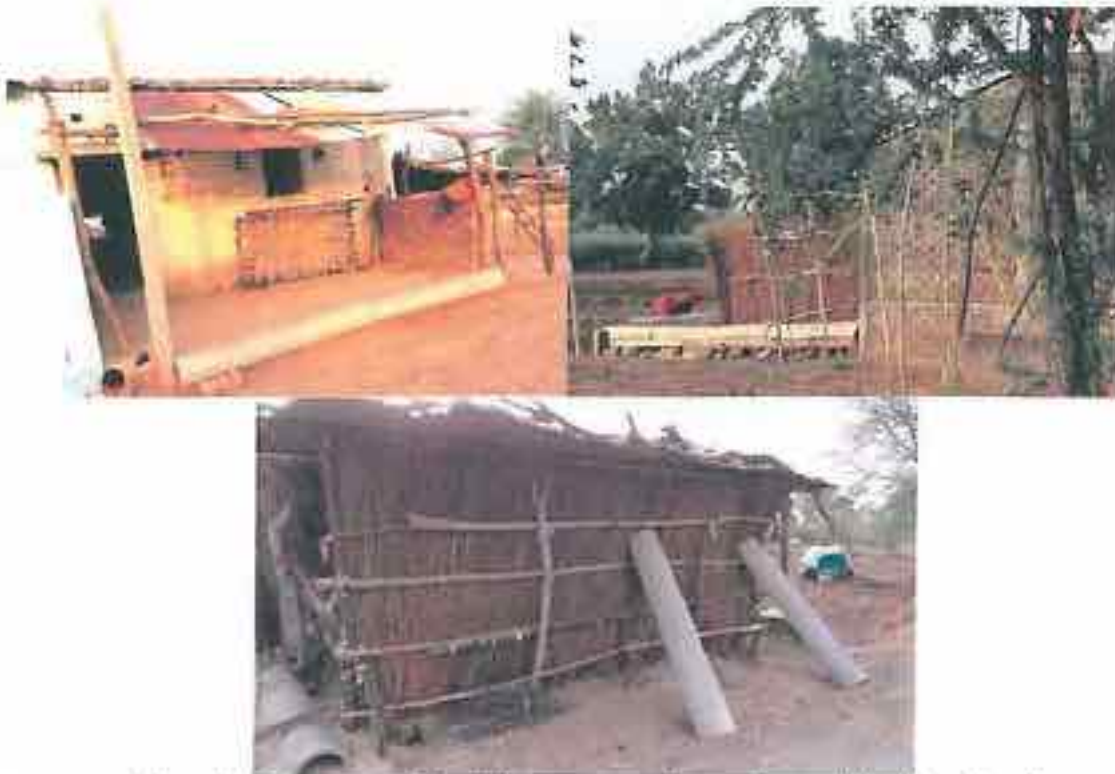
Plate 2.5.10. An opportunity lost in haphazard planning- Case of Brahmangaon
