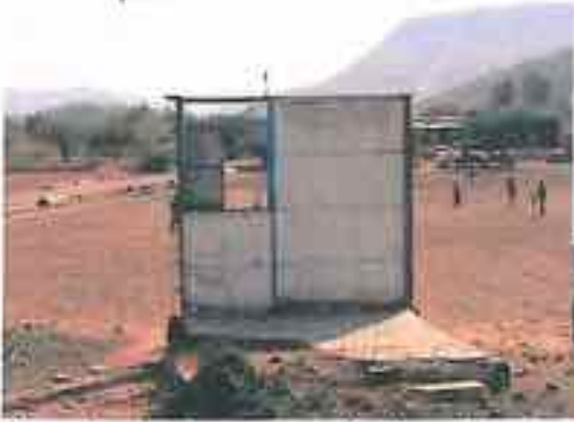
Bhavati - I: Remnants of a Pump House
