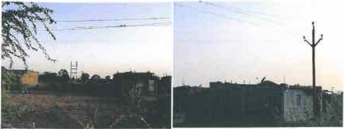
Nimbola: The electric lines need to be relocated.
