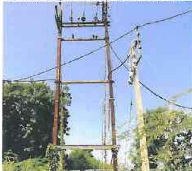
Jalkoti: Only the handle of AB Switch remains
