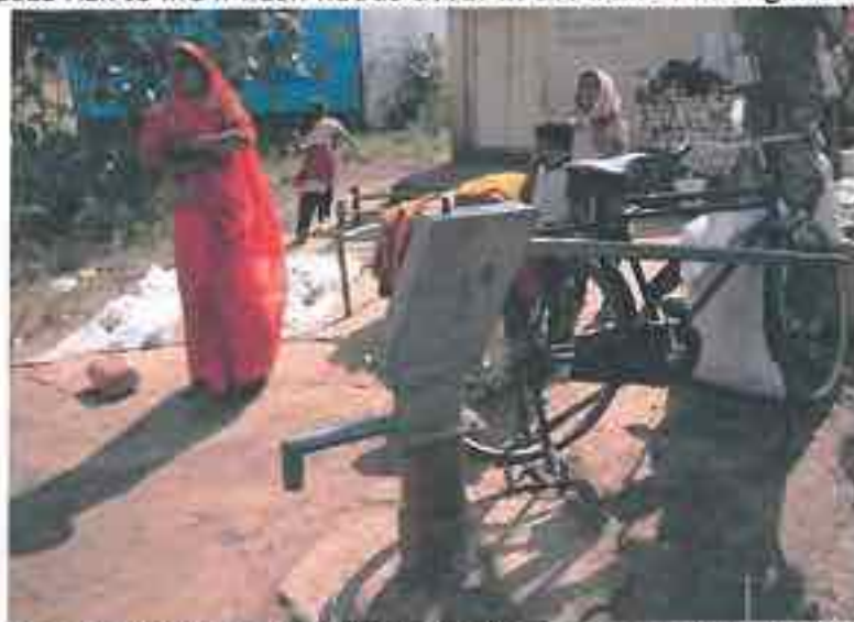
Borlai II: Objectionable HP Location—Right in front of a House. Problem for the Plot owner as public will visit the house at all times, and spills will create havoc and disputes.
