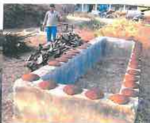
Bhilkheda: Nearby Cistern Platform remains but Cistern is missing
