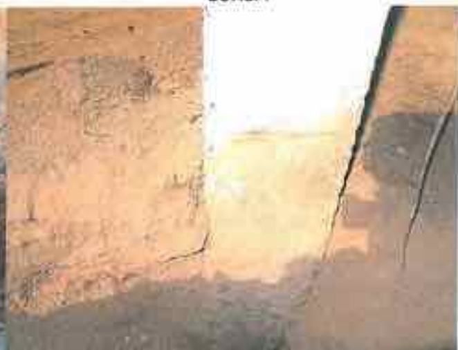
Awalda: No traces of any packing whatsoever
