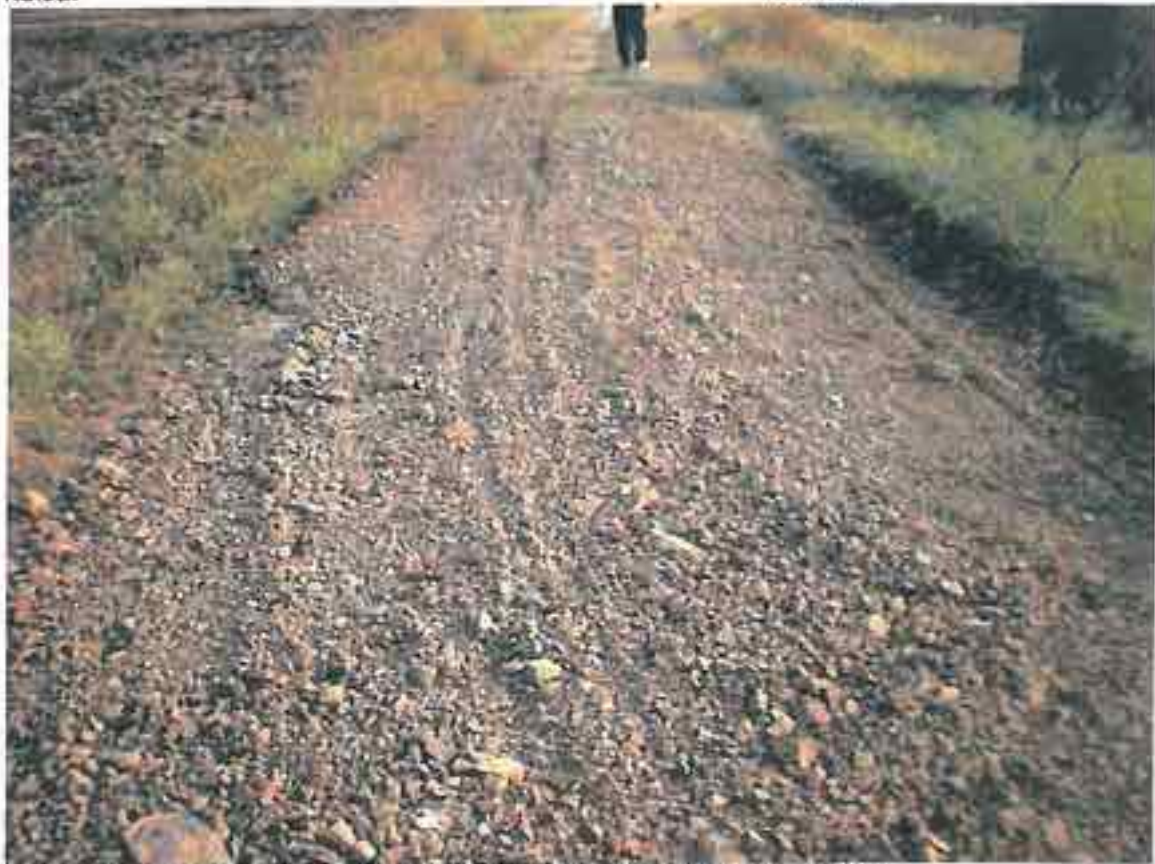
Kaisur : Loose aggregate material, shoulders infested with vegetation.
