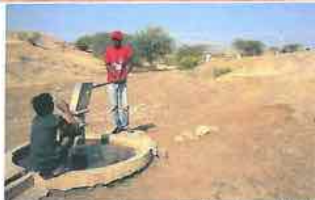
Kikarwas: Two views of the same Handpump. The HP is located in the Nallah trough. This implies likely erosion, flooding in rains, and an inability of people to take water from HP in rains. It also poses risk to life if flash floods occur in the Nallah during monsoons.
