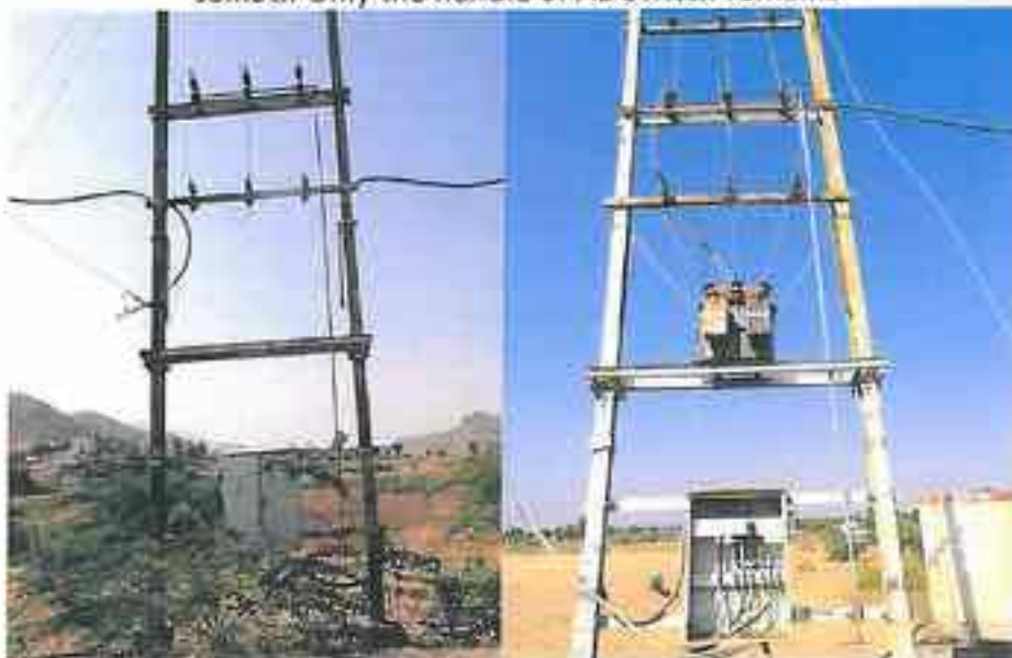
Awalda: AB switches present in two cases-Not a very common occurrence
