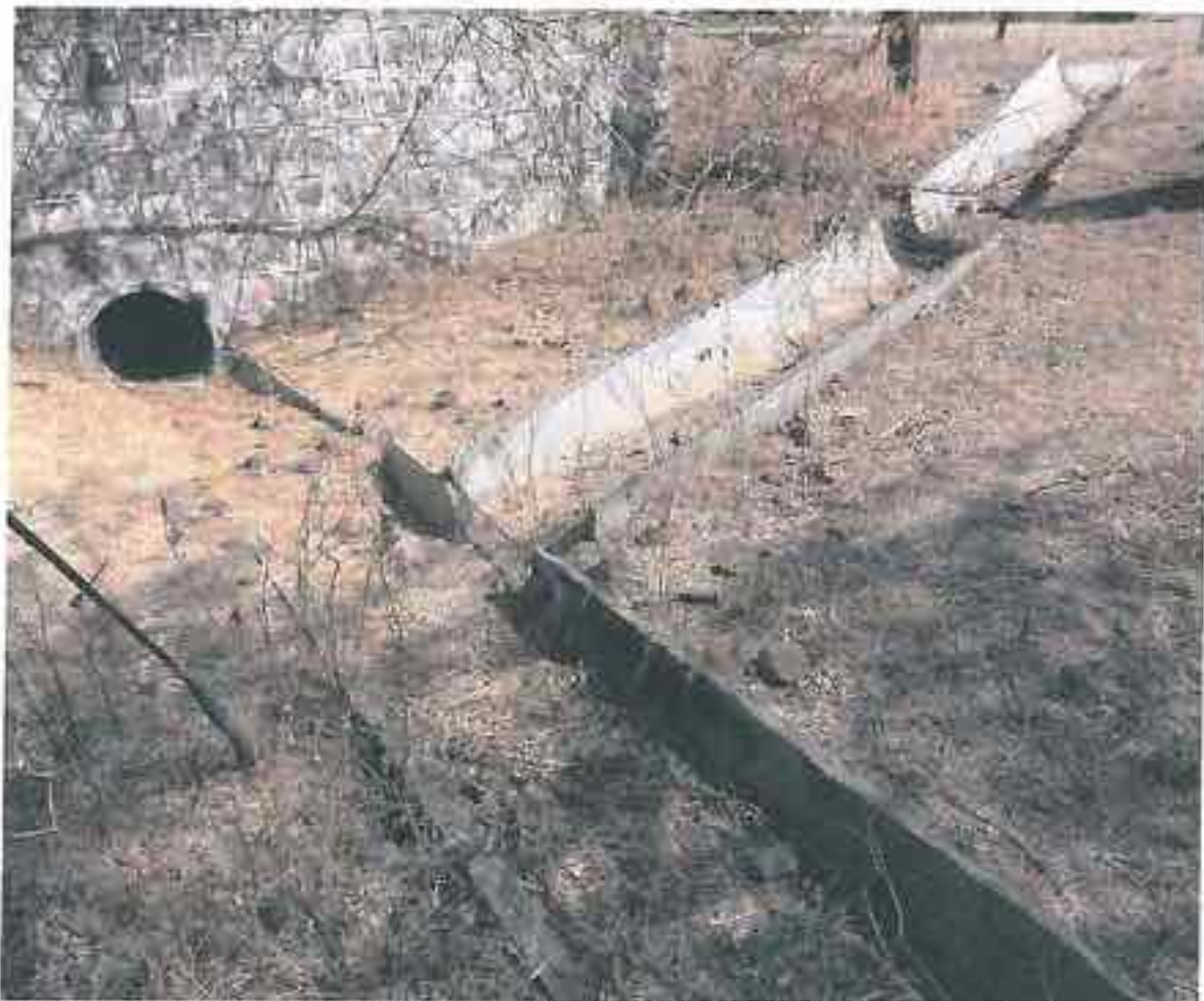
Bhawati II (Typical): Is the outgoing pipe diameter sufficient? Also seen are the broken connections at pipe joints. Two 600 mm half round pipes discharge water into another 600 mm half round pipe.
