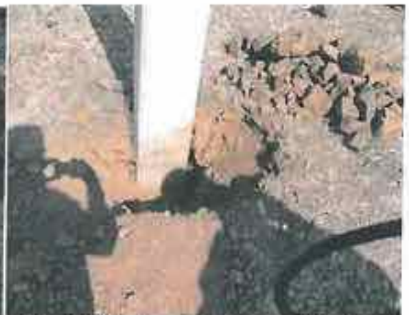
Dehar: Pebbles/aggregate as packing stones
