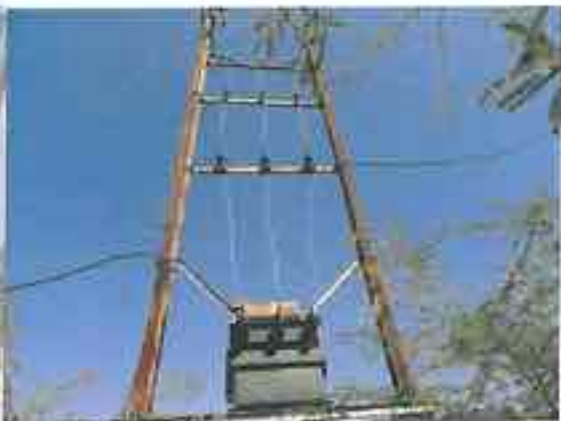
Bijasan: Two Rusted pole, one had remnants of paint work
