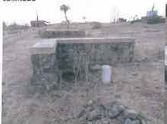
Lohara : plot no 103 in front of culvert mouth
