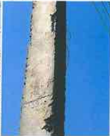
Jalkoti: 3 Poles – poor qualities, missing Paint & external earthing wires wrapped around
