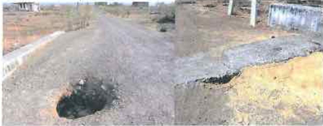
Chichli Kasravad :Massive piping even in hard soil
