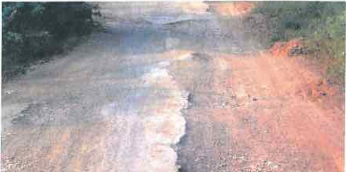
Nisarapur II/III: Distorted road surface
