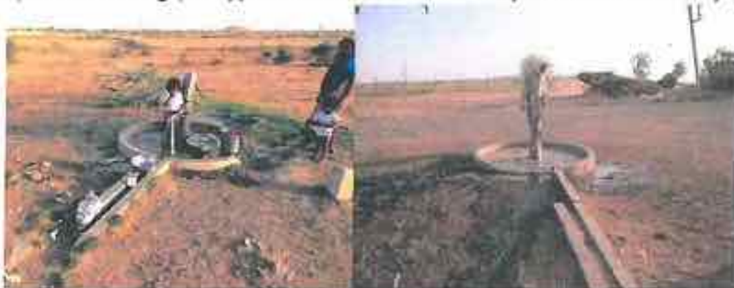
Balkhad: Two different HPs with drainage flow in all directions - the Slope of drainage channel is actually upwards, water finds its own path to drain towards opposite direction. Also, no engineered Approach to the HP seen.
