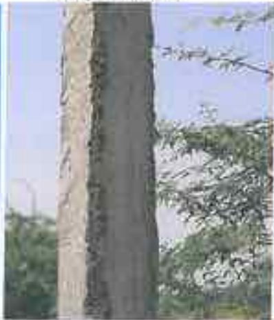
Jalkoti: 3 Poles – poor qualities, missing Paint & external earthing wires wrapped around
