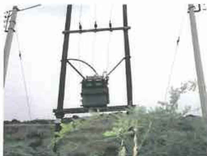
Plate 4.17. Nisarpur: Here even the transformer can be touched, little space left for installing a panel
