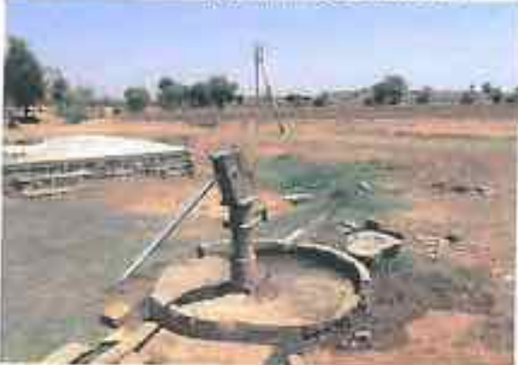
Mandwada: drainage towards road, HP Platform damaged
