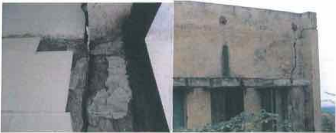
Nisarpur: Men's toilet in Hospital and Primary School building
