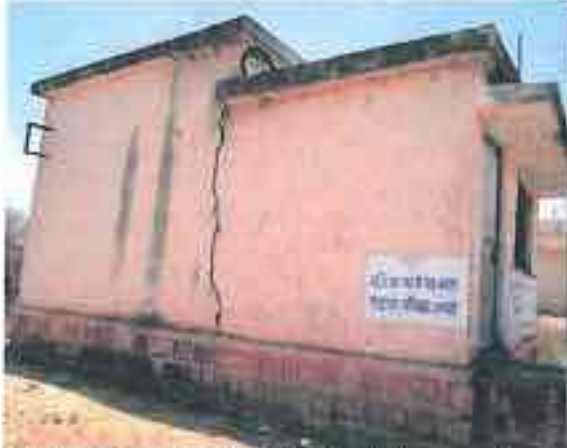
Lakhangaon : Post office Building Khalbujurg: Prominent Cracks Inside School Building. Plate 2.1.1 Typical Damaged buildings at various R&R Sites .....cont....
