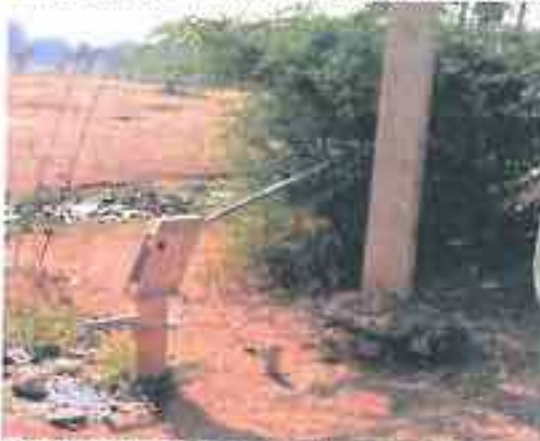
Kalyanpura: electrical pole prevents operation
