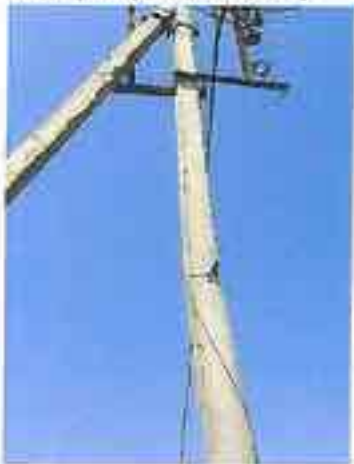
Jalkoti: 3 Poles – poor qualities, missing Paint & external earthing wires wrapped around
