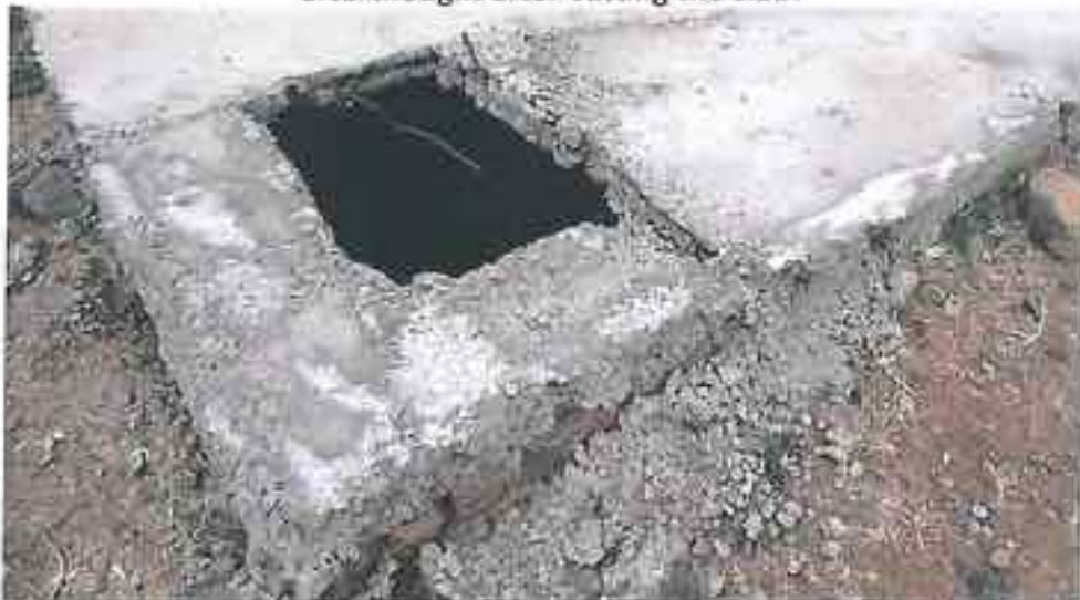
Barda Manavar: No outlet seen. Post-construction correction in the form of inspection/maintenance opening. The construction carried out later as a patchwork is itself is of very poor quality, not likely to last. Noticeably, Bricks are visible in the new part.
