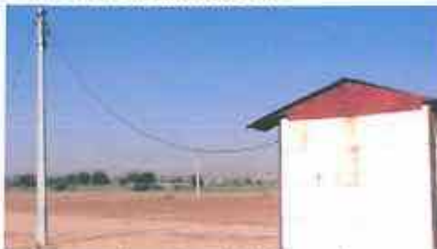
Separate electric line laid for pumphouse.
