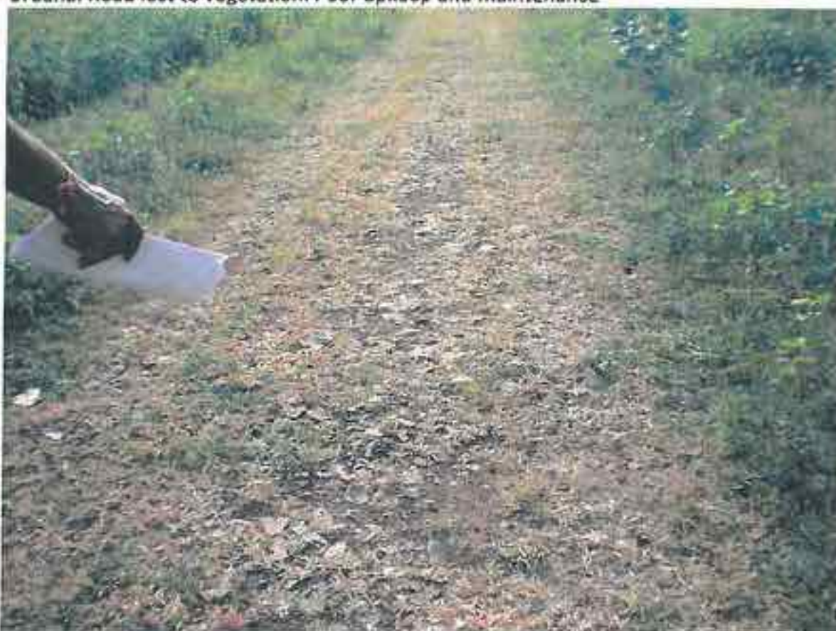
Khajuri, Jhabua: Road lost to grass and vegetation
