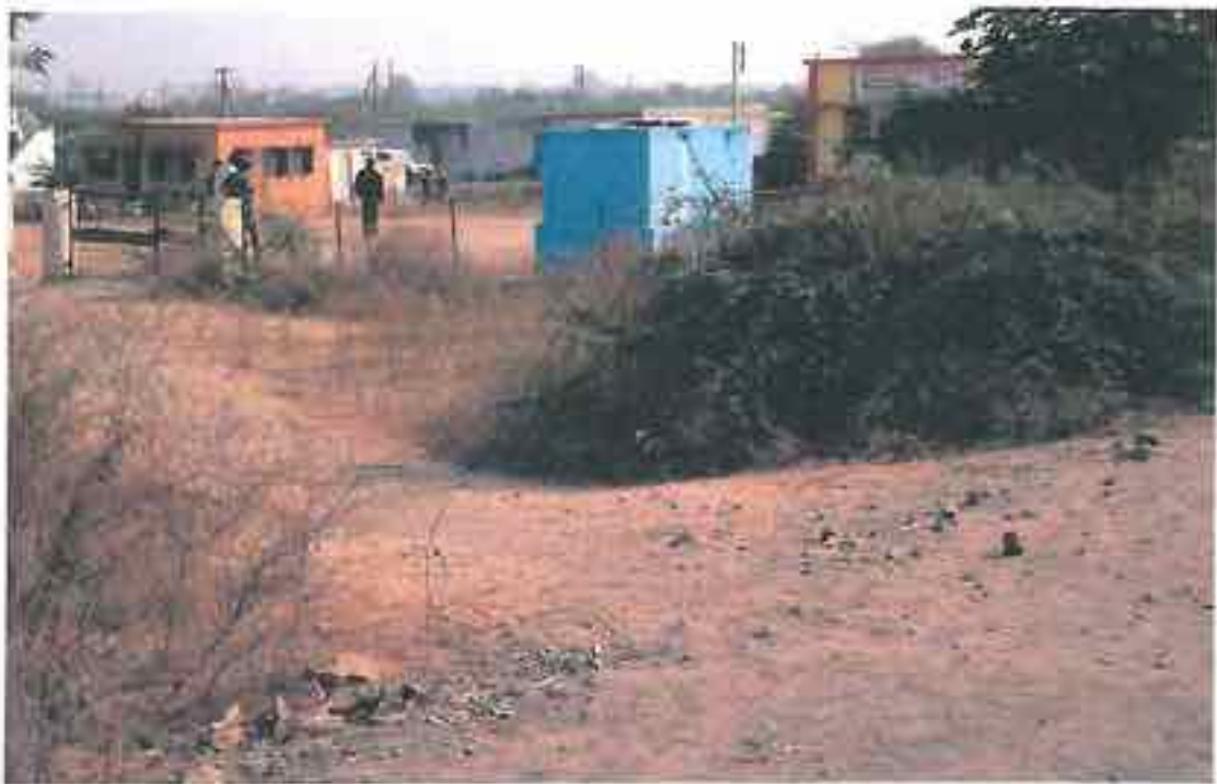
Kukra: Lack of smooth entry to the buildings. The road could have been extended a few meters to reach the gate (or better till the school building), but this small patch has been left undeveloped without considering likely problems during Rains.
