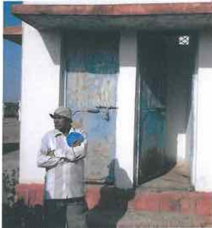
Kavanthi: One of the toilets is locked
