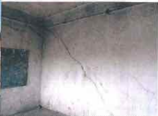
Lakhangaon : Post office Building Khalbujurg: Prominent Cracks Inside School Building. Plate 2.1.1 Typical Damaged buildings at various R&R Sites .....cont....
