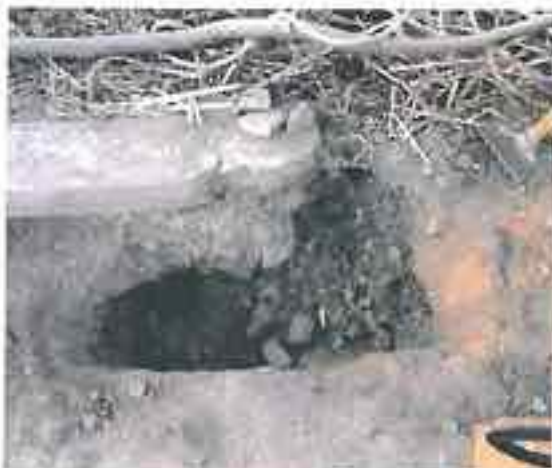
Sirsani: No trace of pack around a fallen pole
