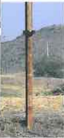
Borlai II(Phase II): Year 2011 construction, and yet the paint is missing
