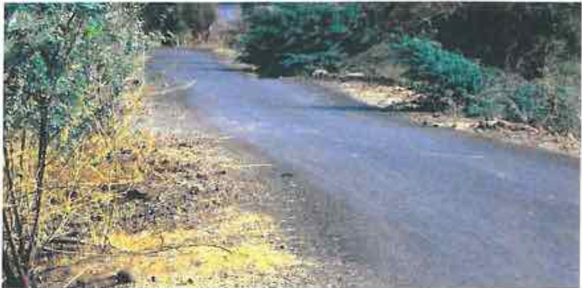
Moreghadi: Undulating, Wavy Road Surface.
