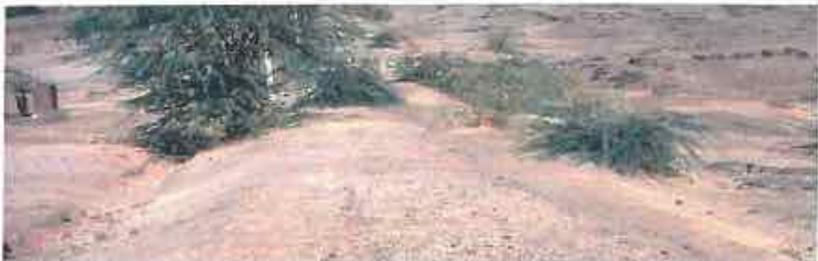
Morekatta: Poor roads, dilapidated shoulders, and lack of maintenance of roads indicated by growth of bushes.
