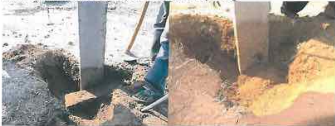
Plate 4.28. Morekatta: (Left) Readily available Plot marking stone stacked in pole base, (Right same pole after removal of this marking stone – No semblance of packing below
