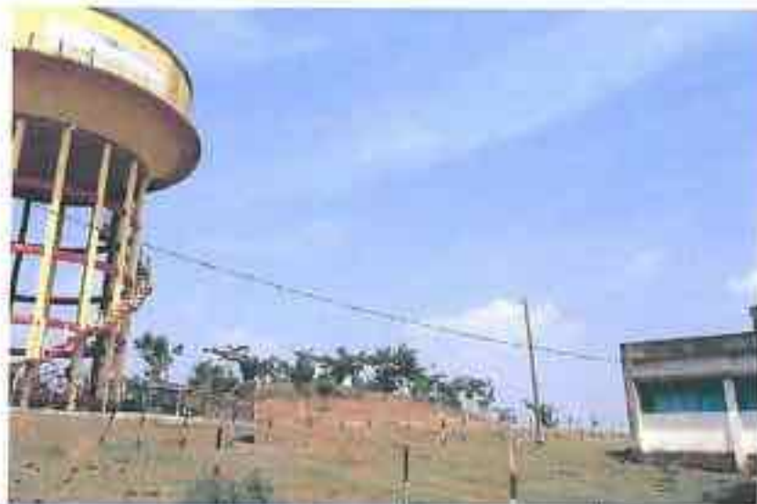
Nisarpur: scour/sluice valve discharges water to highway, crossing which it would enter hospital.
