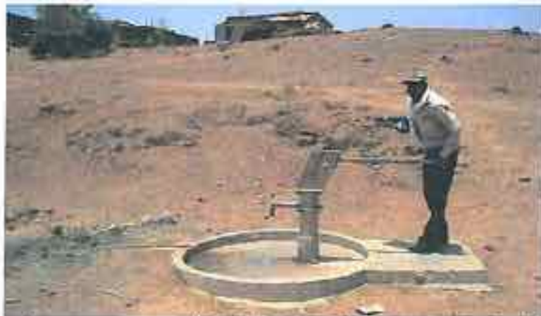
Chenpura: No drainage, no approach-Residents need to carry water load all the way up
