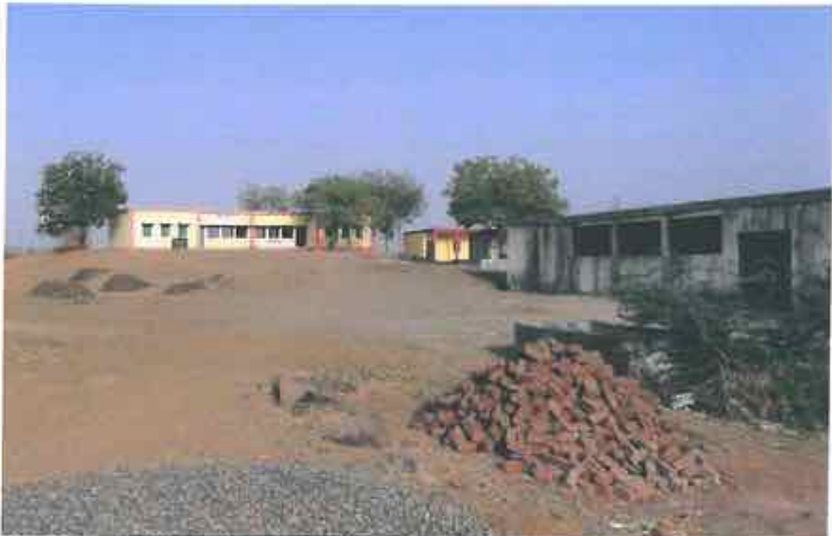
Plate 4.44. No Electric lines in the near vicinity of Middle School building at Datwara. Classes expected to run without fans and lighting.
