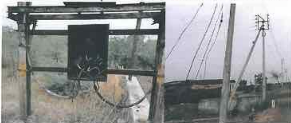
Dharampuri: Pole placed on Culvert
